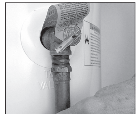
Figure 16 - The T&P Relief Valve discharge pipe must be installed properly and piped to an adequate drain.
