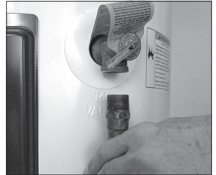
Figure 13 - Removing the T&P Relief Valve discharge pipe.
