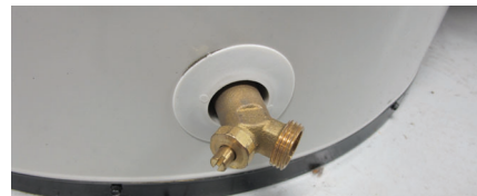
Figure 33 - Drain Valve
